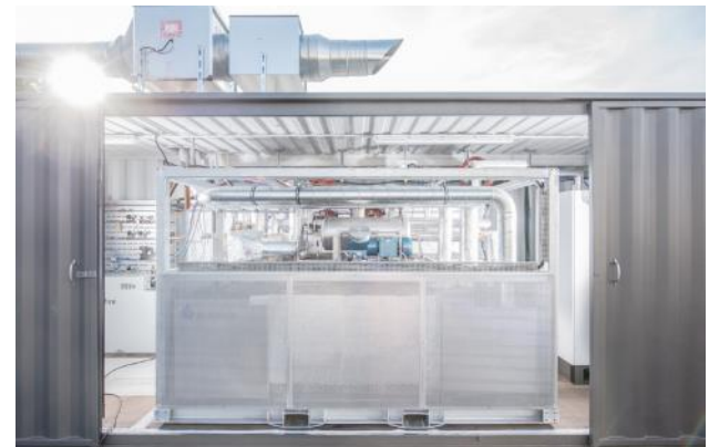
System testing in Dresden
